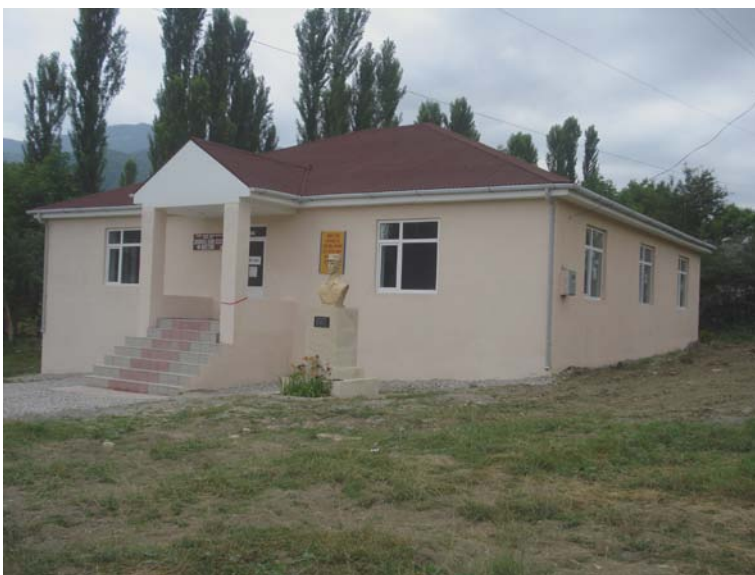
And this is Khanagah village school constructed through allocations of Japanese Embassy for AZN 69 thousand
