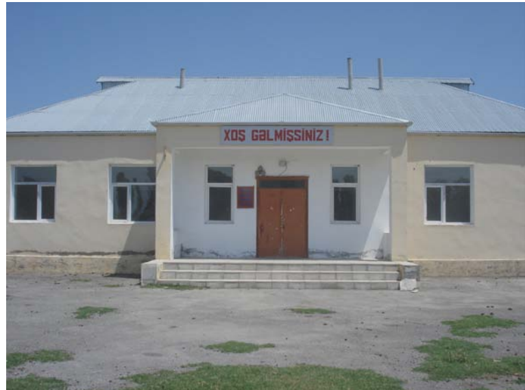
This is Garabagi village school of Khachmaz region, constructed through state budget funds of AZN 149 thousand in 2007.
