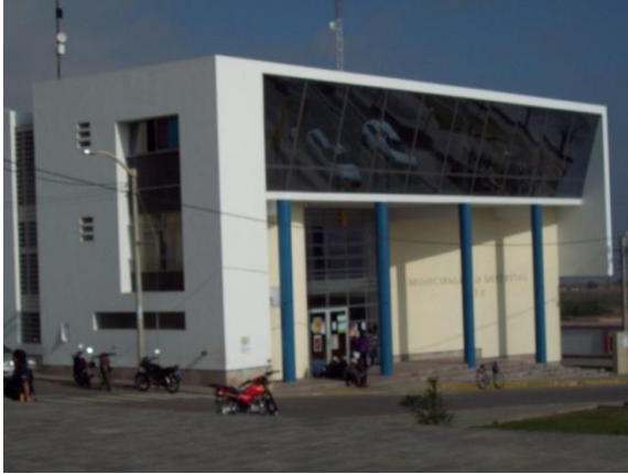
The new municipal building in Ite now at risk of collapsing.
